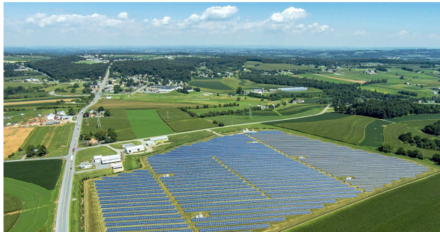
.5-3 MW Merchant Generator/Community Solar
